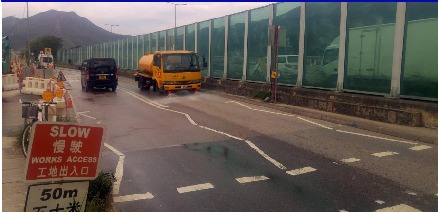
Road surface cleansing along Tai Wo Service Road West
