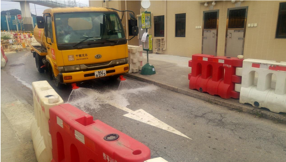
Figure 3 – Water Spray for Active Construction Area
