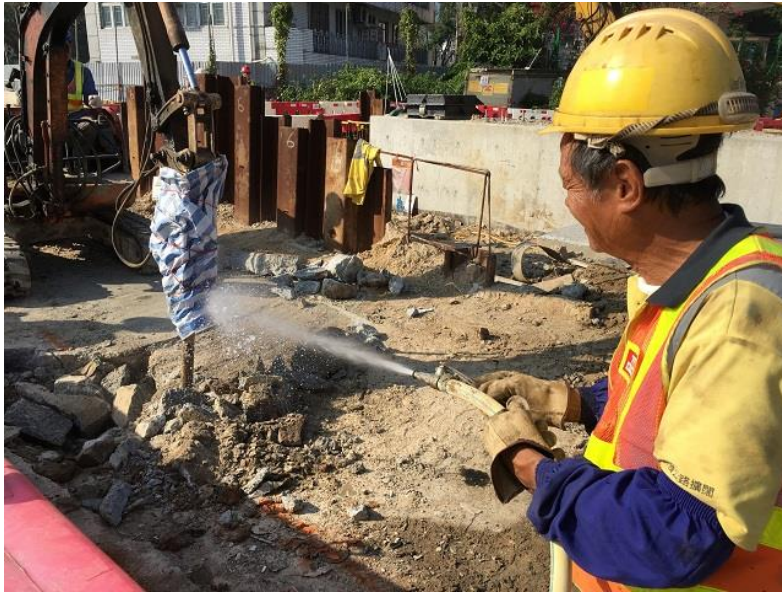
Figure 5 – Water Spray for Dust Emission Construction Activity
