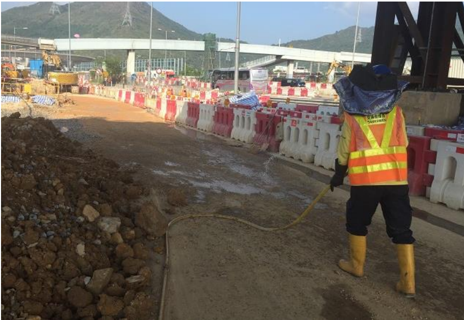
Figure 3 – Water Spray for Active Construction Area
