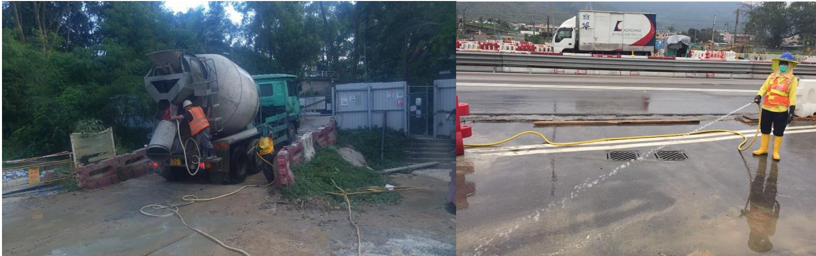
Figure 4 – Wheel Washing Facility at Exit Point
